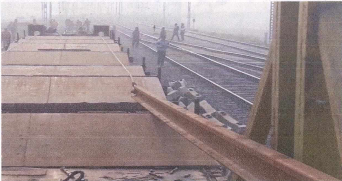
First Rail tied to track through chute
