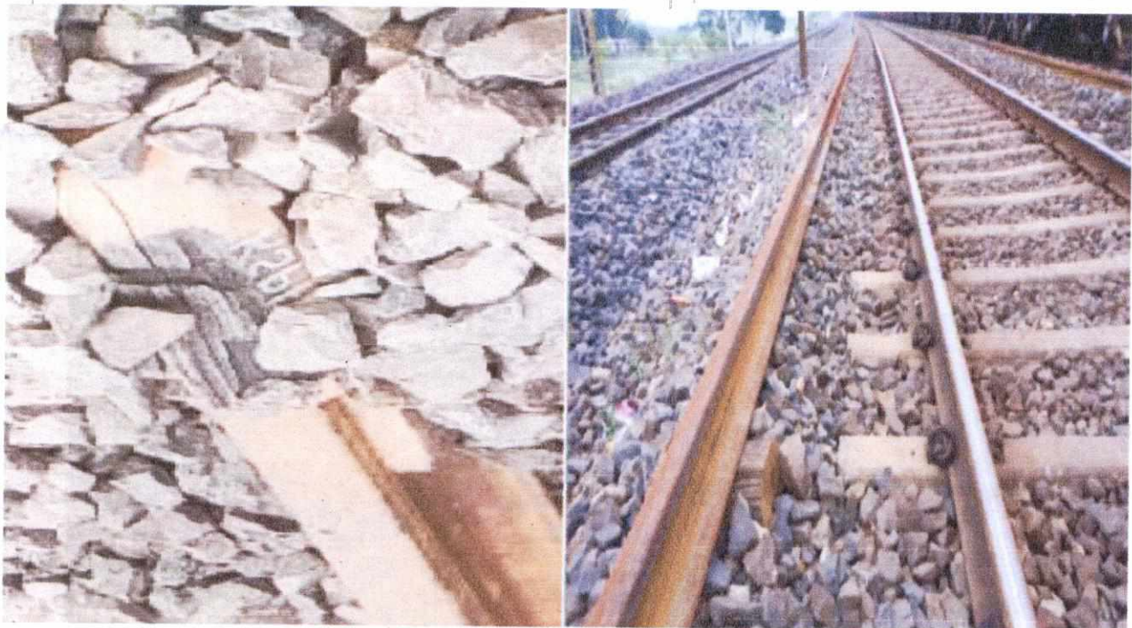
UNLOADED RAILS PROTECTED BY GUTKA
